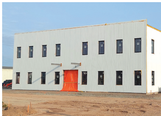
Brunswick Lift Rental (Ferdinand)
