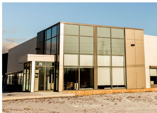
Foulem Construction (Rufin)
