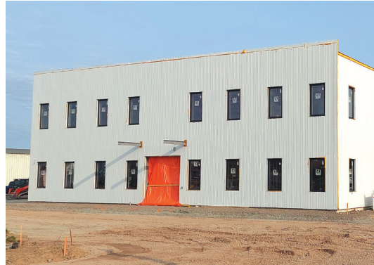
Brunswick Lift Rental (Ferdinand)
